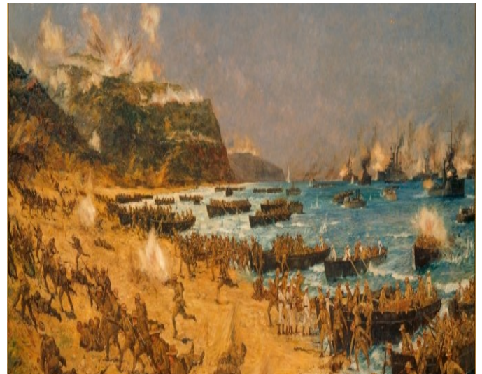
Anzac Cove Landing 25 April 1915
